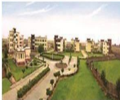
JAGANNATH UNIVERSITY, Village Rampura, Tehsil Chaksu, Jaipur (Rajasthan)
